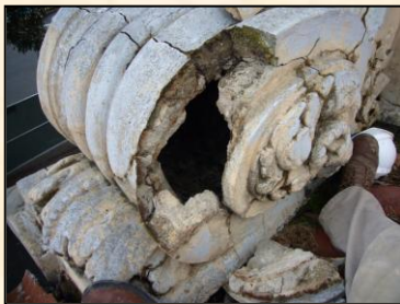
Realigning top, replacement of loose pieces with pins, and crack repair
