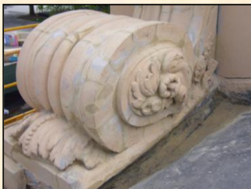
Reinforcement of loose pieces with pins, and crack repair
