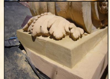
Composite patching with Jahn M70, and crack repair
