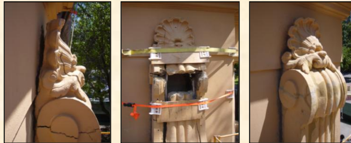
Realigning top, replacement of loose pieces with pins, and crack repair
